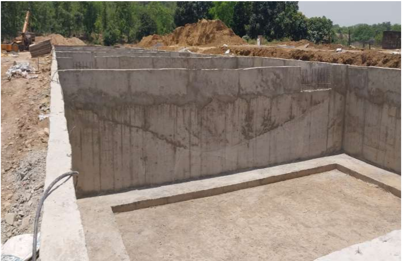
Settling Tank & Thickner for Waste/Effluent Water Treatment to ensure ZLD
